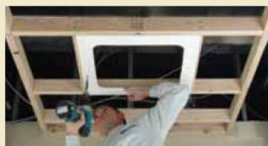
2. Mount Stealth surround with drywall screws.
