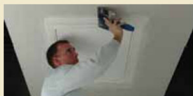
4. Tape and apply drywall compound.
